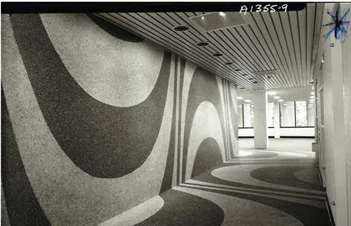
Figure 2.21 Patterned, exposed aggregate finish to floor and wall in lift lobby of entrance foyer to rear (seven-storey) block of offices. Also shows original metal deck ceiling lining and downlights (undated and unattributed). (Source: Rick McEwan, Lipman Constructions files)
