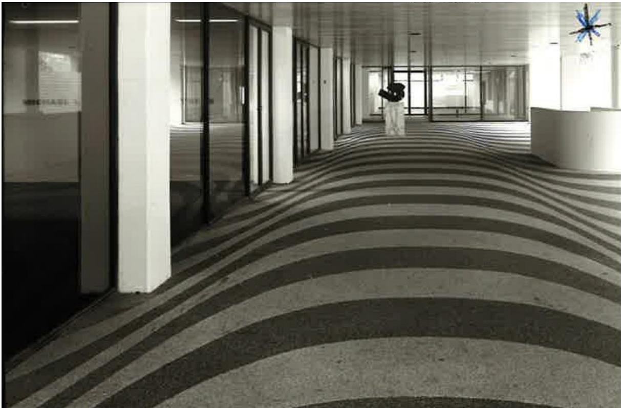
Figure 2.20 South colonnade with patterned, exposed aggregate finish to concrete floor and Clement Meadmore sculpture in front of entrance foyer to rear (seven-storey) block of offices (undated and unattributed). (Source: Rick McEwan, Lipman Constructions files)
