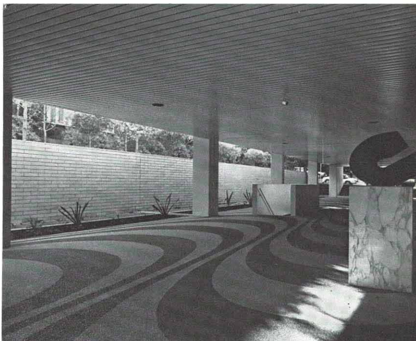
Covered entrance concourse to 41 McLaren Street with a flamboyant curving floor design of reconstructed stone paving.
